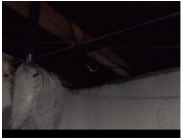
Visible image basement wall penetration.
