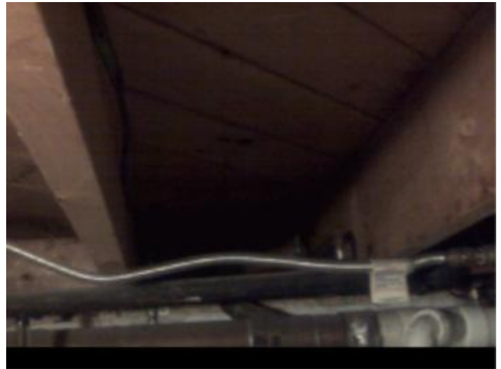
Visible Image of rim and band joist.
