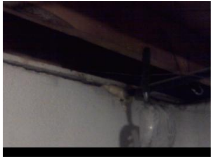
Visible Image of plumbing wall penetration.
