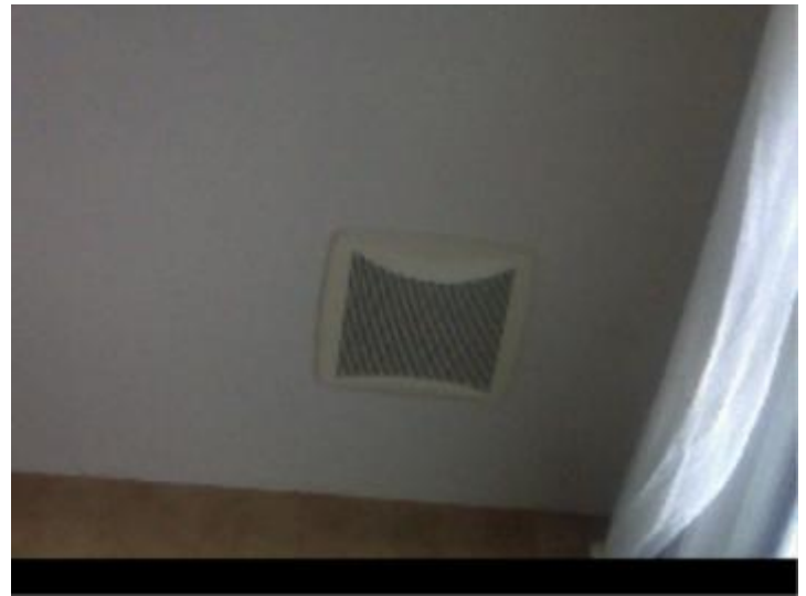
Visible image of ceiling vent.
