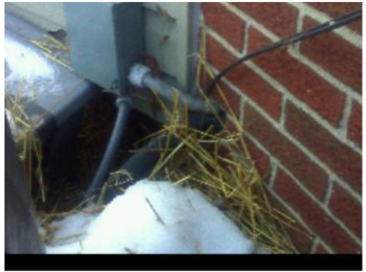
Visible Image of Electrical wall penetrations.
